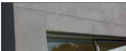
Figure 2.7.1 Neat finish of horizontal joints
